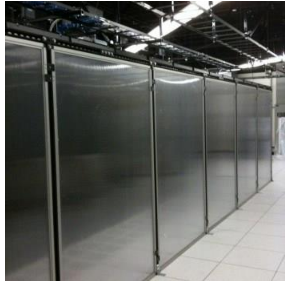
DAMAC cold aisle containment
