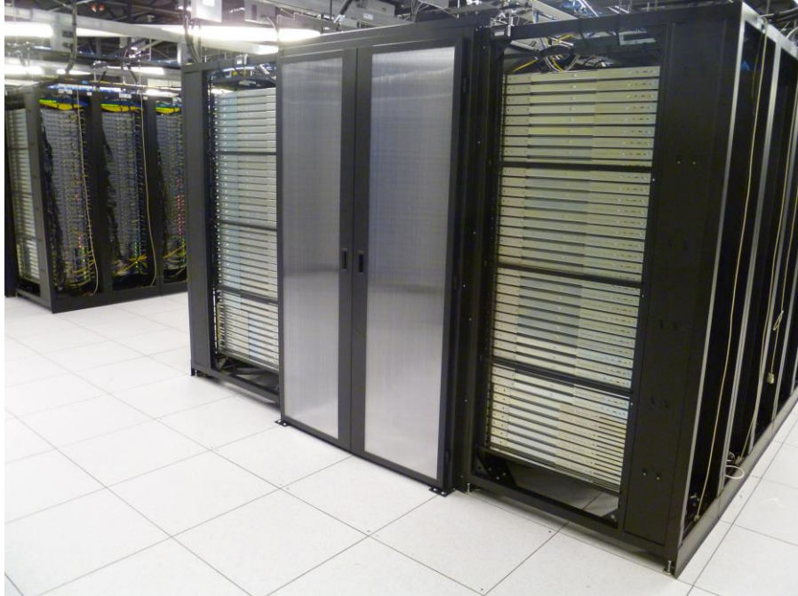
DAMAC cold aisle containment
