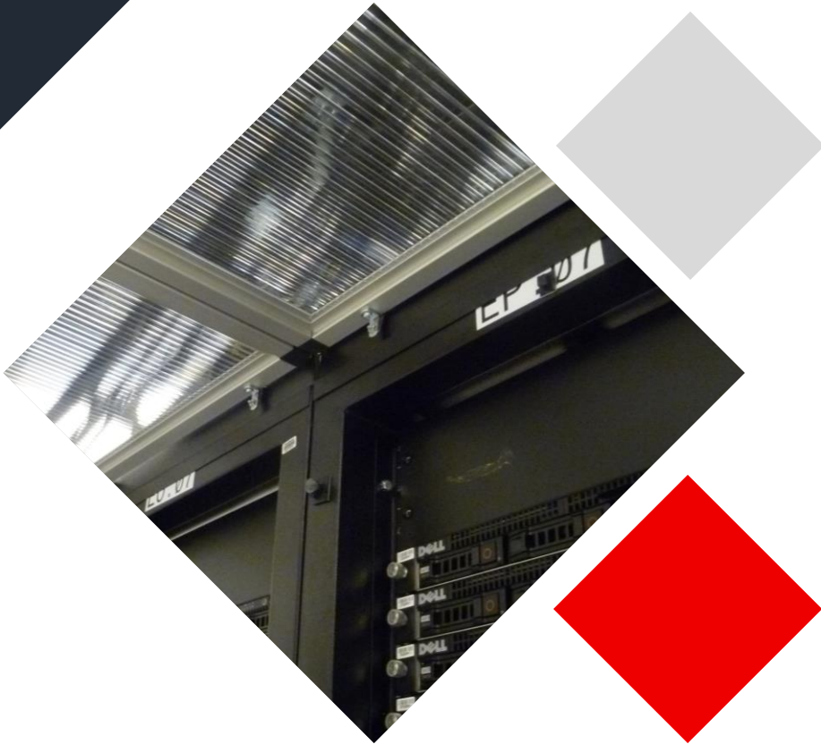
DAMAC hot aisle containment
