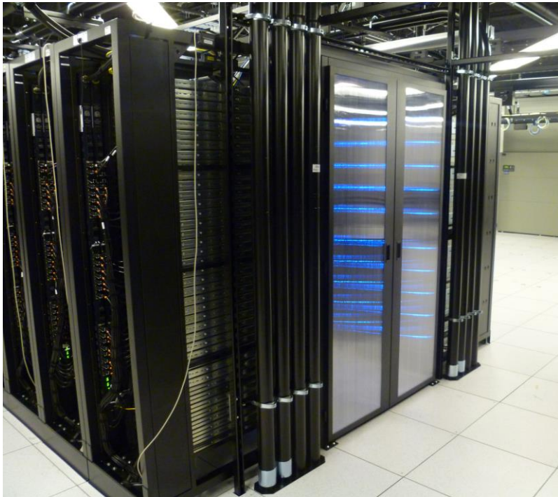
DAMAC cold aisle containment
