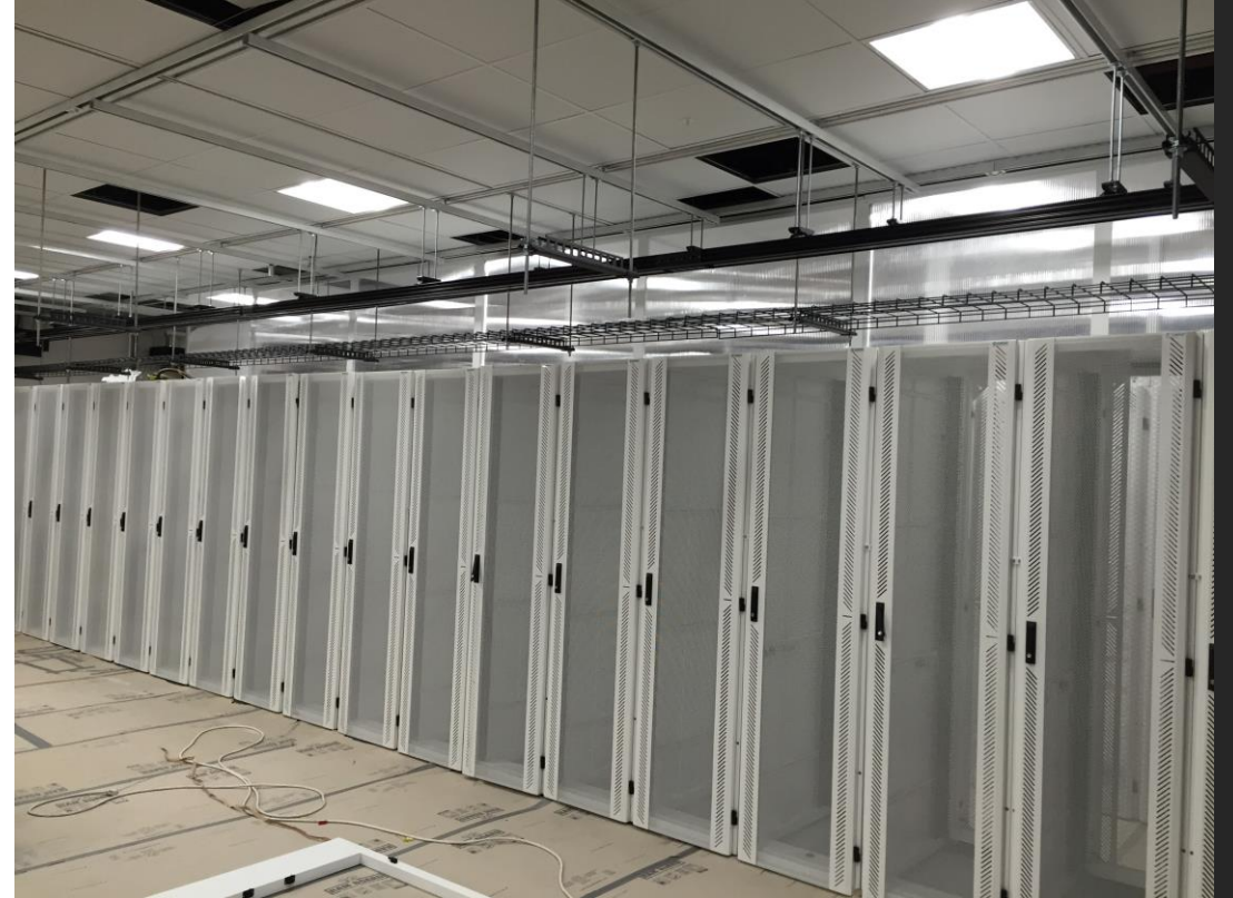
DAMAC cold aisle containment
