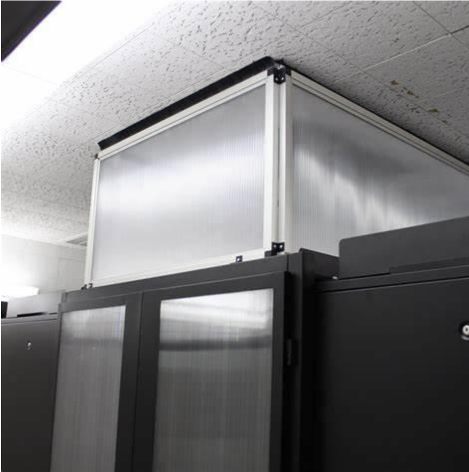
DAMAC hot aisle containment
